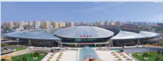
BEIJING SOUTH STATION
